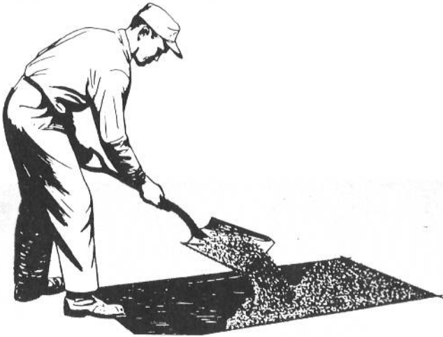
Placing plant-mix in cut
